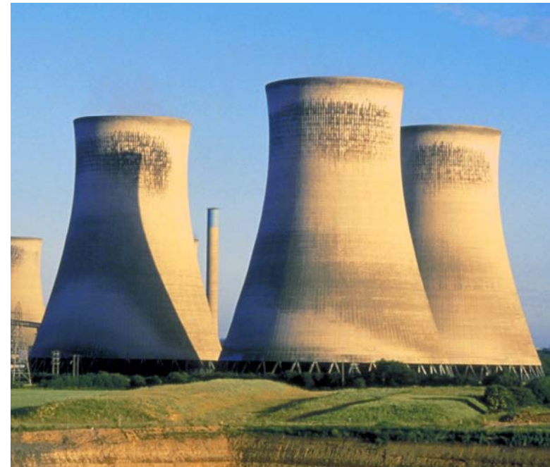
Cooling towers keep the core of a nuclear power plant at a safe temperature.
